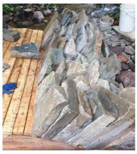
The project was to guild a dry stone bridge across Salem Creek with an over water span of about 8 feet and an overall length of about 30 feet for the bridge.
