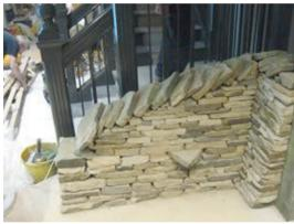
frames or lines. The wall went together well with a corner being built, then the wall tapering down in line with the staircase. The wall was topped off and the finishing touch was a brass Yorkshire Dry Stone Walling Guild plaque fixed to the last top stone at the bottom of the stairs.
