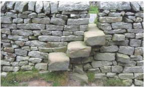
As you go through a new gate you will notice what looks to be a new wall running across the field. The wall end to the left has not been built very well as there are a lack of runners going into the wall. You will then cross through several gates and keep your eyes left to see a good example of a cripple hole. These were built into the walls to
